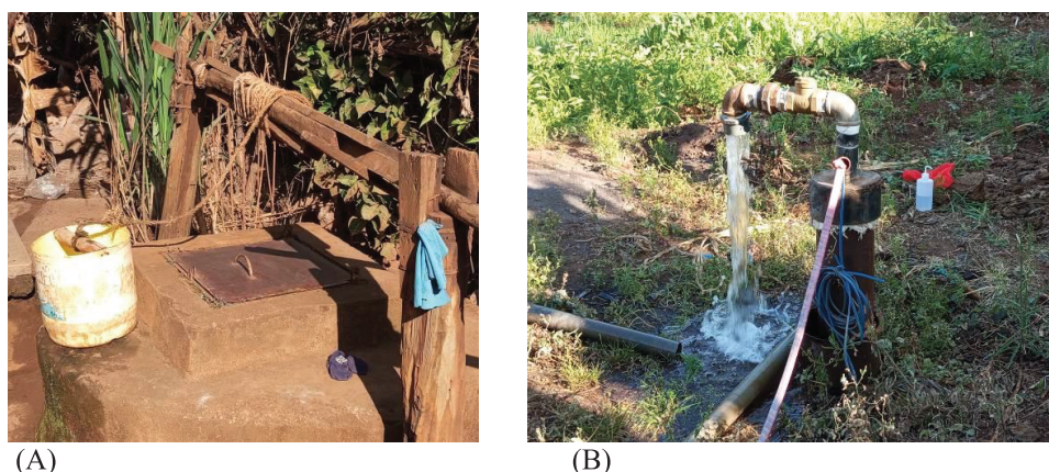
Fig. 2. (A) Boreholes B10 (hand-dug well <10 m deep) and (B) B19 (drilled tube well >50 m deep) in Imenti Central and Tigania East sub-counties, respectively.
